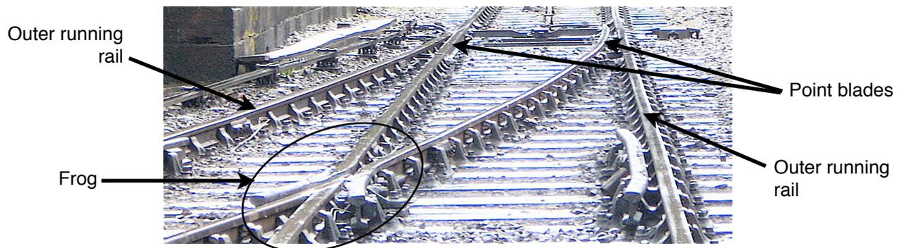
pointwork. However, they also complicate wiring. A live frog turnout comprises three electrical elements. Two are the outer running rails. The third is everything else - the frog and the rails connected to it, as well as the point blades. As the points change, the frog becomes electrically connected to one or other of the outer running rails according to which one the blades touch. The *polarity* of the frog is said to change.
